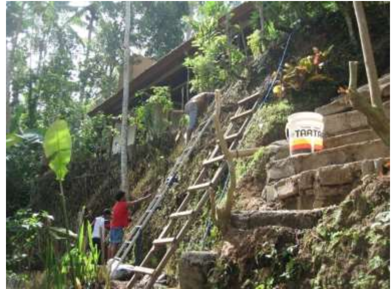
Planting vetiver using long ladders
