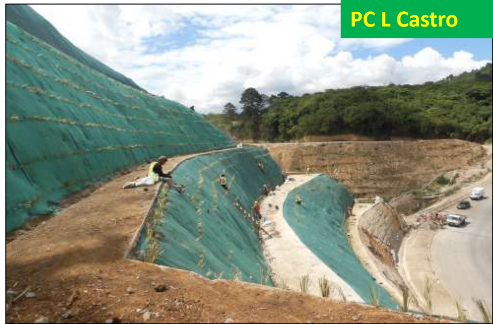
Very steep Batters with geofabrics
