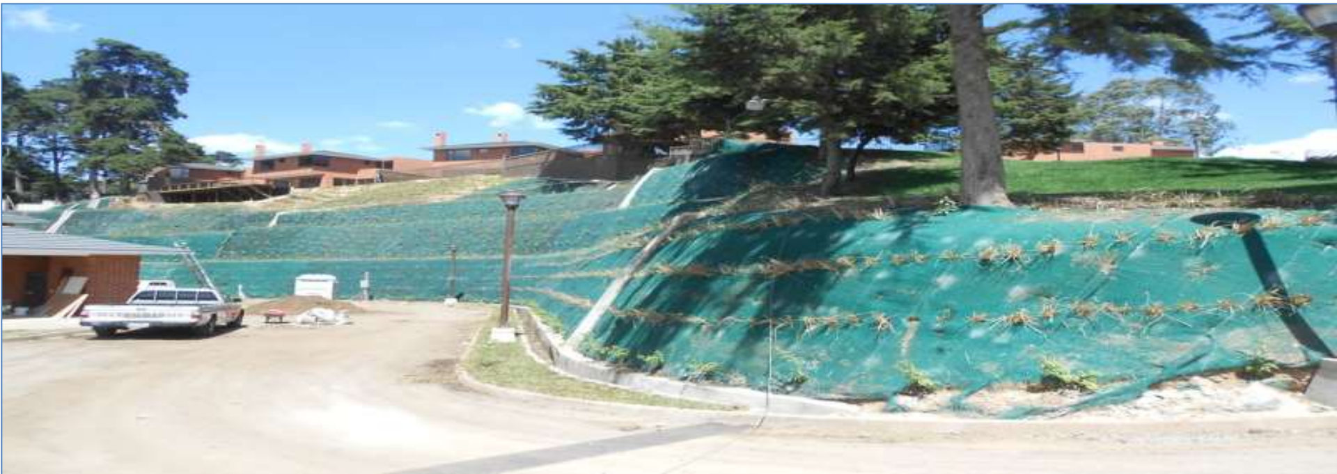
Very steep Batters with geofabrics
